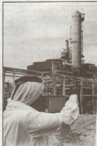
Qatar refinery at Umm Sai
